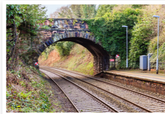
stone railway bridge
