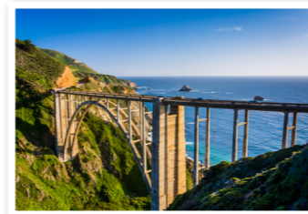
concrete road bridge
