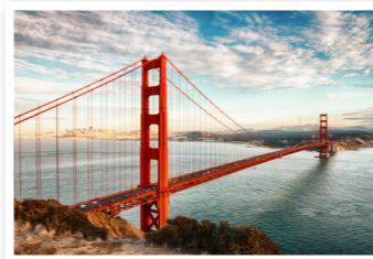
metal suspension bridge
